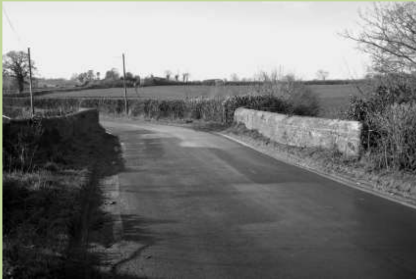
SALKELD BRIDGE OVER THE RIVER DIVILISH
