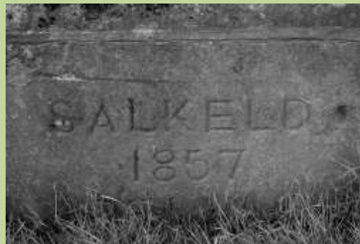
INSCRIPTION ON LEFT SIDE OF BRIDGE (PARTLY OVERGROWN)
